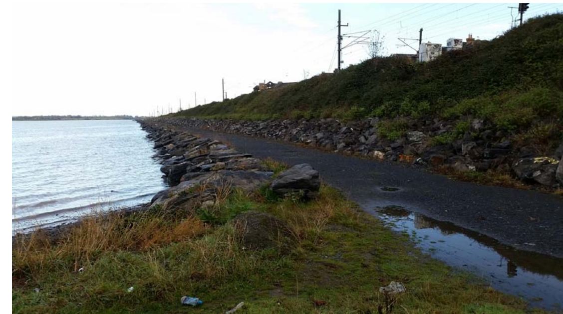
PHOTO 1 - EXISTING WEIR MAINTENANCE TRACK
