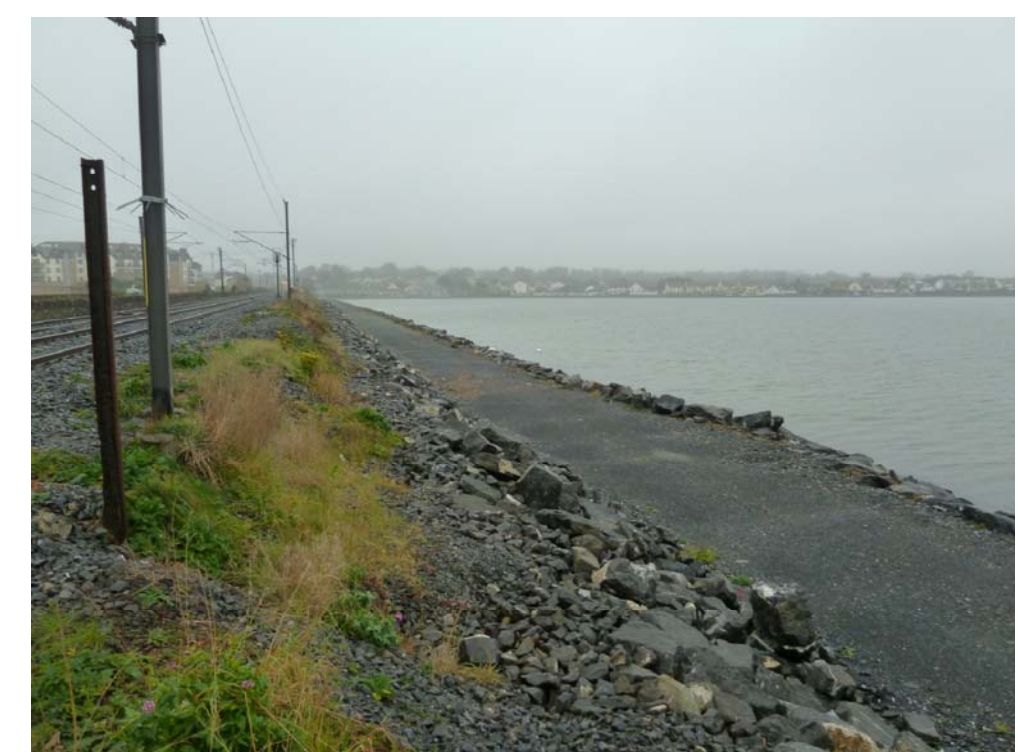
PHOTO 2 - EXISTING WEIR MAINTENANCE TRACK
